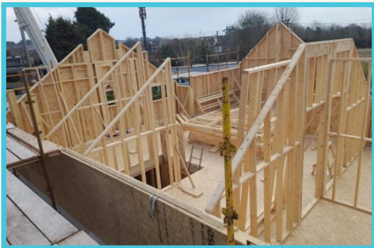
Figure 6: Timber frame building being erected.
