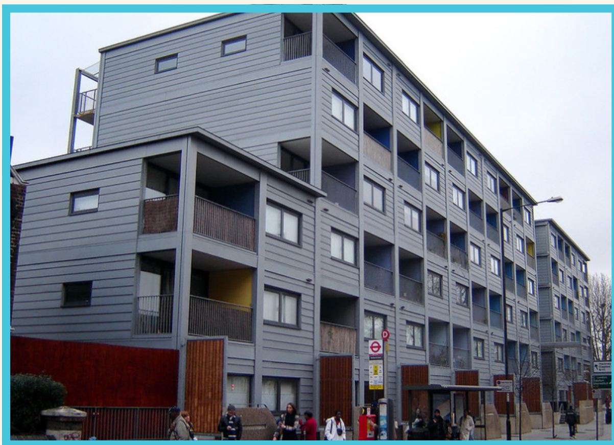
Figure 2: Modules stacked on a completed building.
