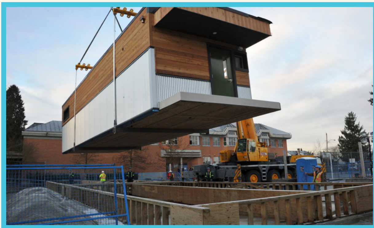
Figure 1: Module being hoisted onsite.
