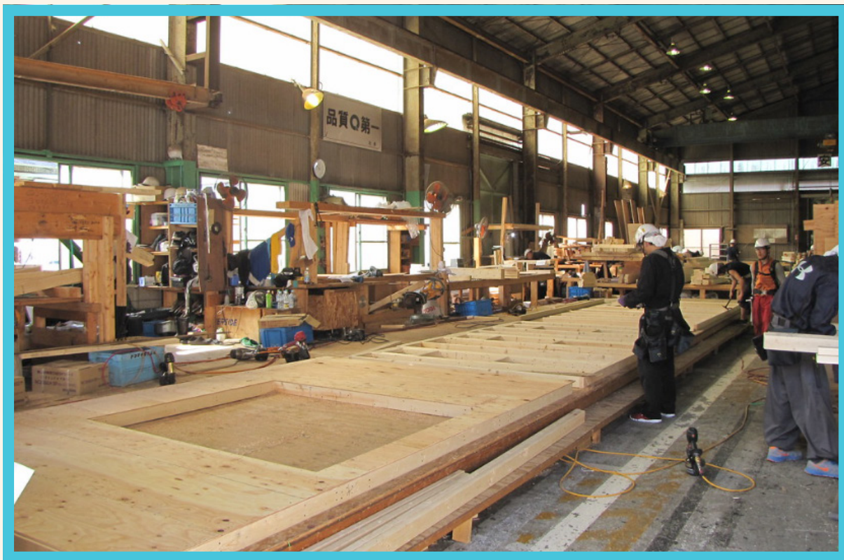
Figure 5: 2-D panel being built in a factory.
