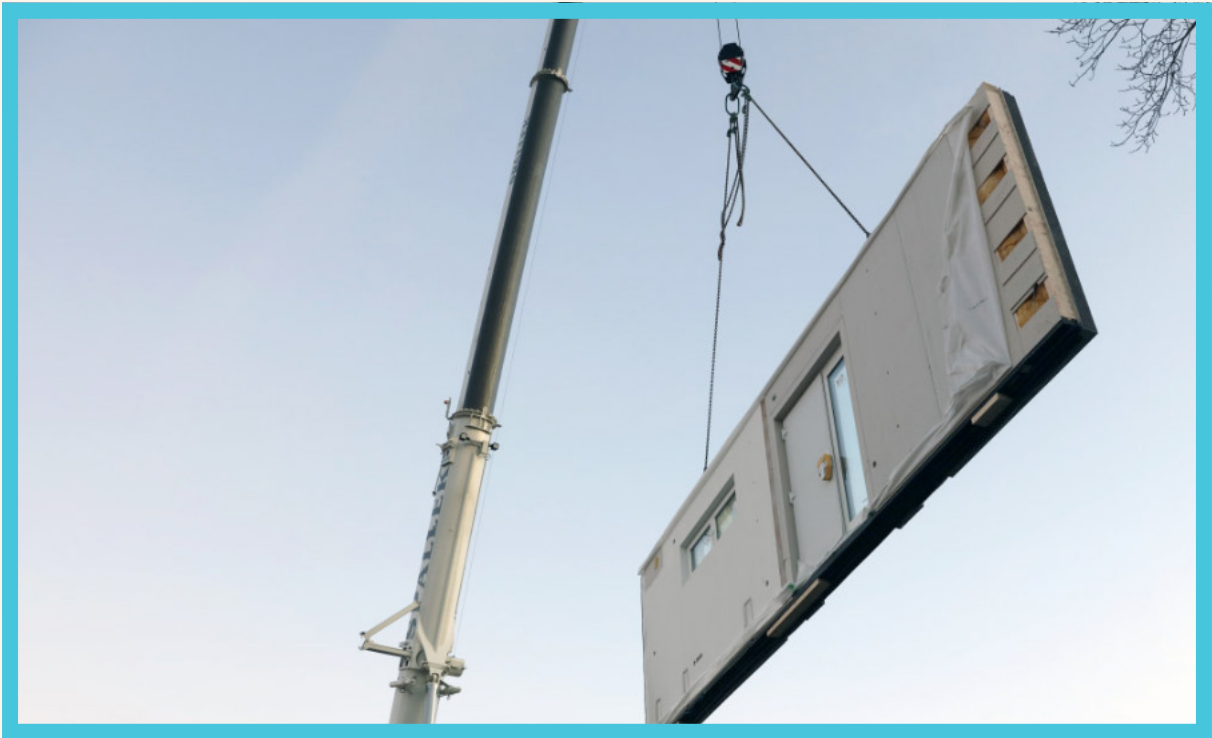
Figure 3: 2-D panel being hoisted onsite.
