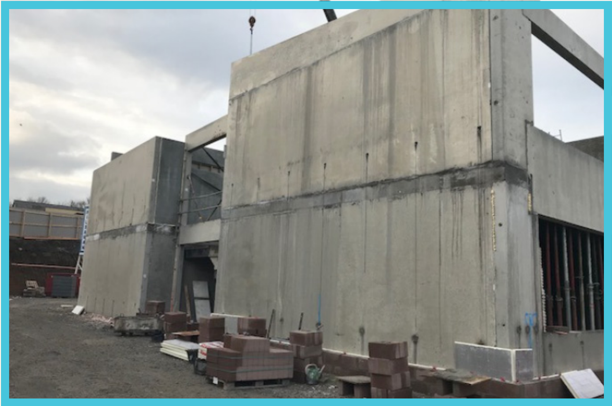
Figure 4: 2-D precast concrete walls being assembled.
